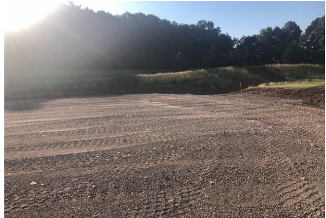
Crushed Material Placed – Bus turn-around
