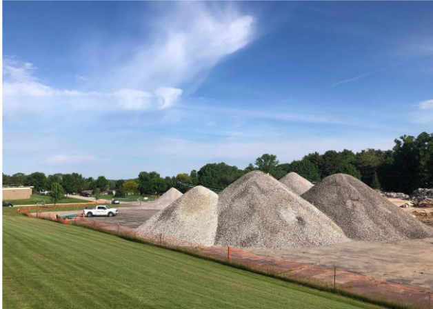
Crushed Vacant Building Material Stockpile
