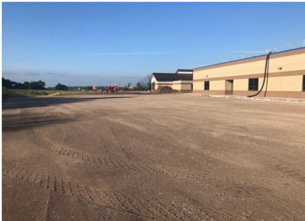
Crushed Material Placed – Bus turn-around
