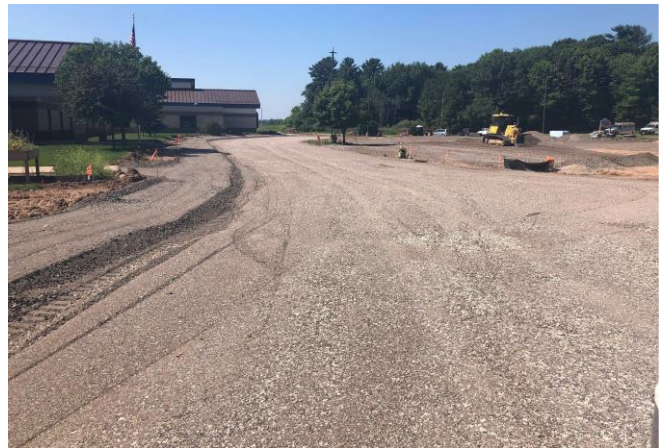
Crushed Material Placed – Front Drive/Parking
